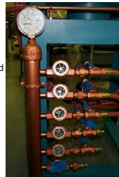
Photograph of closed loop system with common dial flow indicators and flowtek switches.
