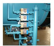
Photograph of closed loop system with Malema flow sensors and integrated flow indicators.
